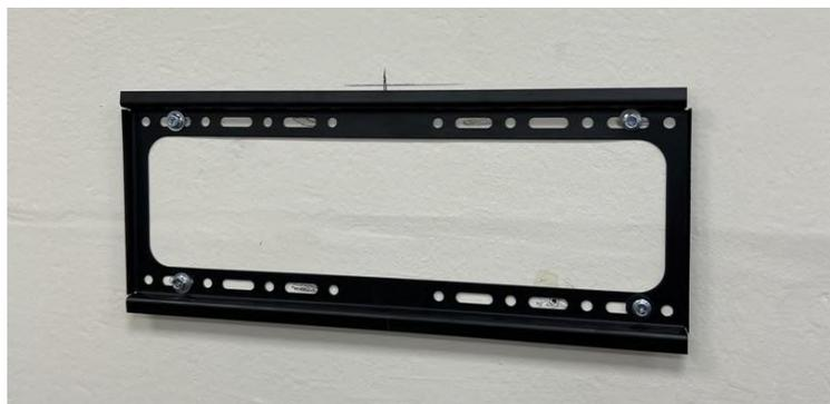
Now pick your screen up and attach any cabling that is required. After doing so, reattach the security covers. A second person could be helpful at this stage.
