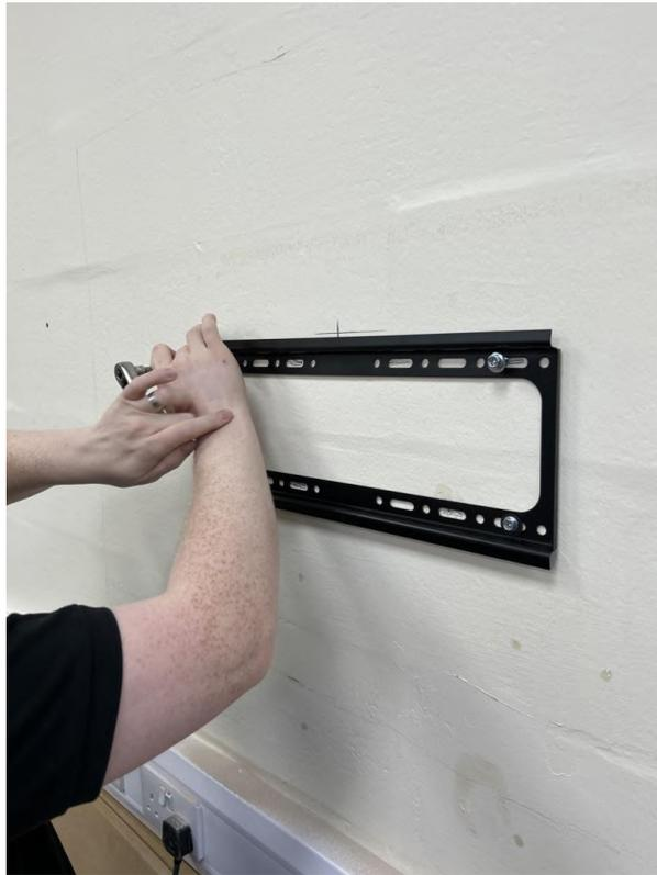
Once you have created your holes, you will need to insert the plugs provided. Next, line up your mount and begin to screw it into the plugs. Please note: do not fully tighten any screws until all are inserted.
